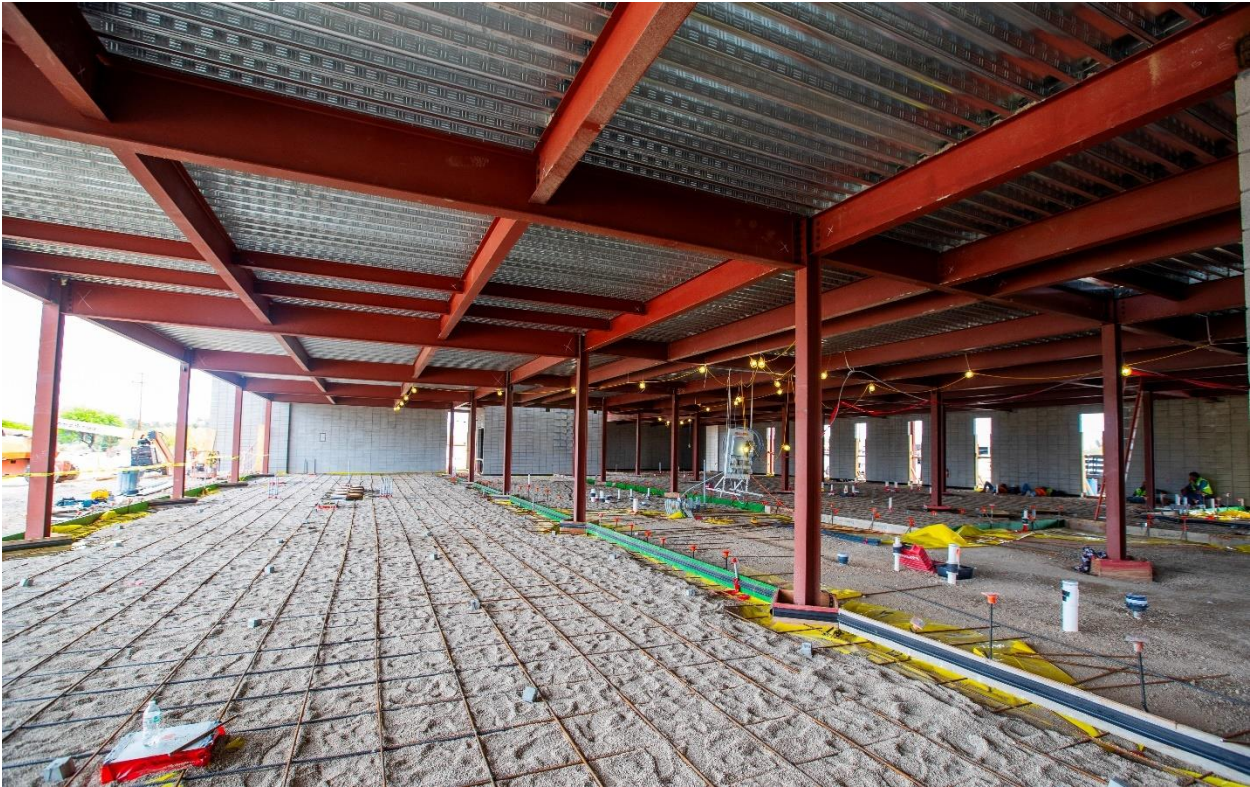
First Floor Interior Progress
