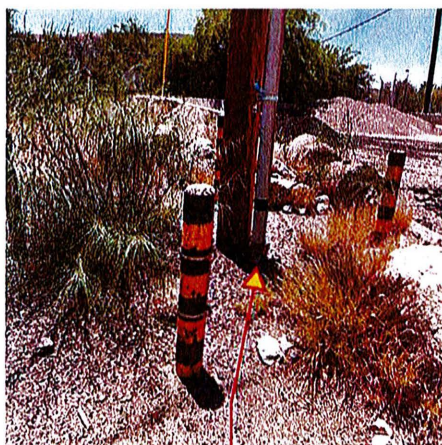
TEP POLE WITH RISER TO PIMA COUNTY VAULT
