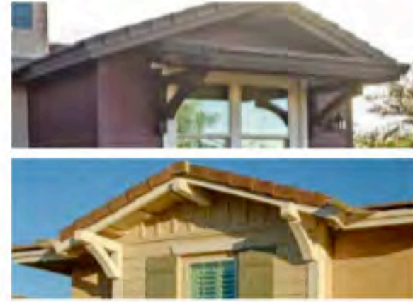
2. Gable End Window Detail with Corbels
