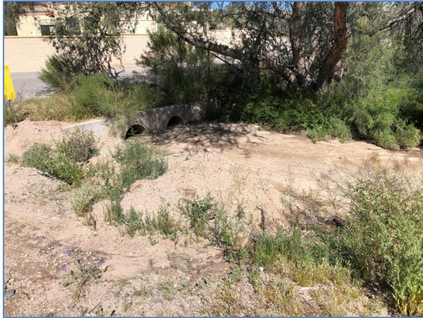
Photo 4 - Sediment compromised culvert at La Cresta & Overton roads
