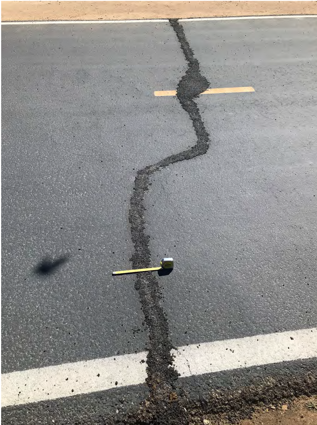
Loop Path System past half way toward La Cholla Blvd, typ larger crack, recently patched
