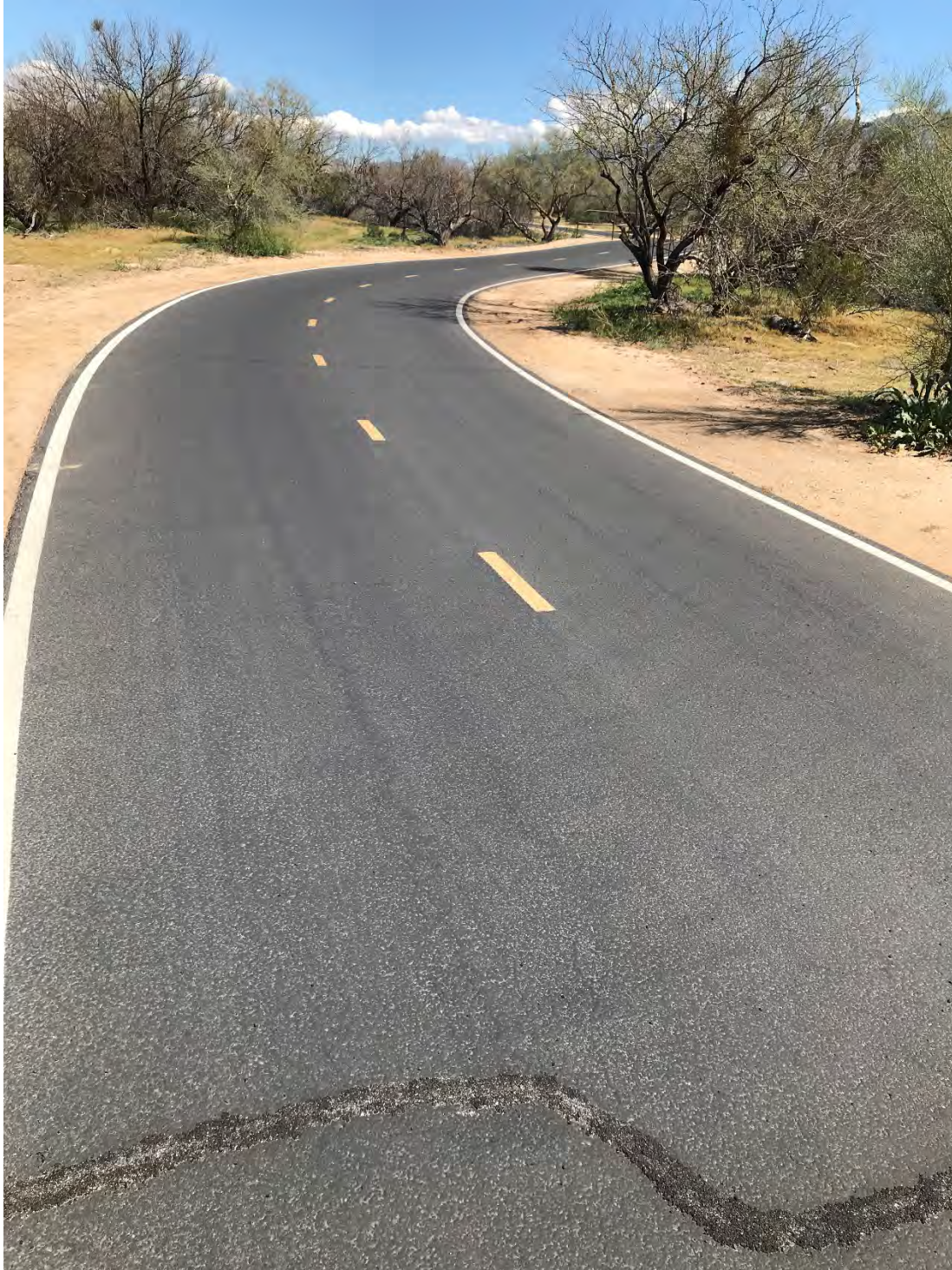
Loop Path System past half way, looking back toward La Canada Dr, note typ crack frequency
