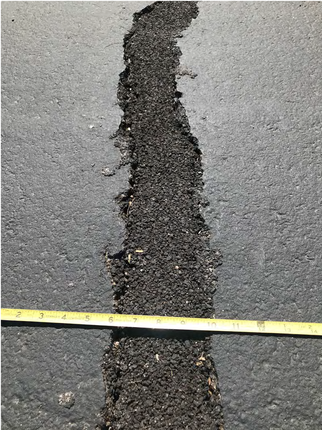
Loop Path System near La Canada Dr – travelling back toward La Cholla, note displacement At 4" a little larger than typical avg of about 2' to 2.5"
