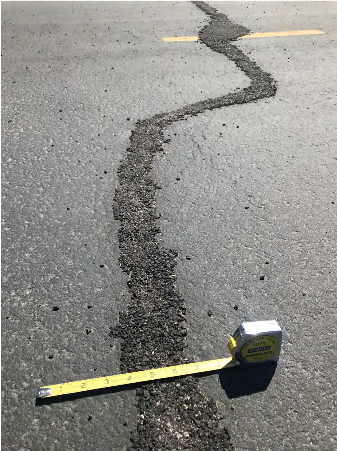
Loop Path System past half way toward La Cholla Blvd, typ displacement at ~ 2.5"
