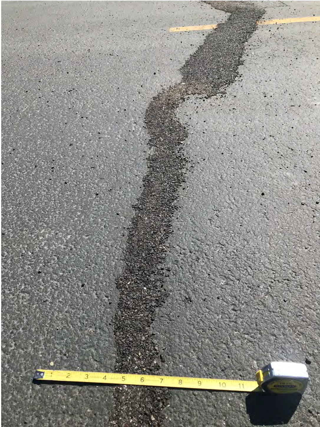
Loop Path System approaching La Cholla Blvd, typ displacement of recently patched crack
