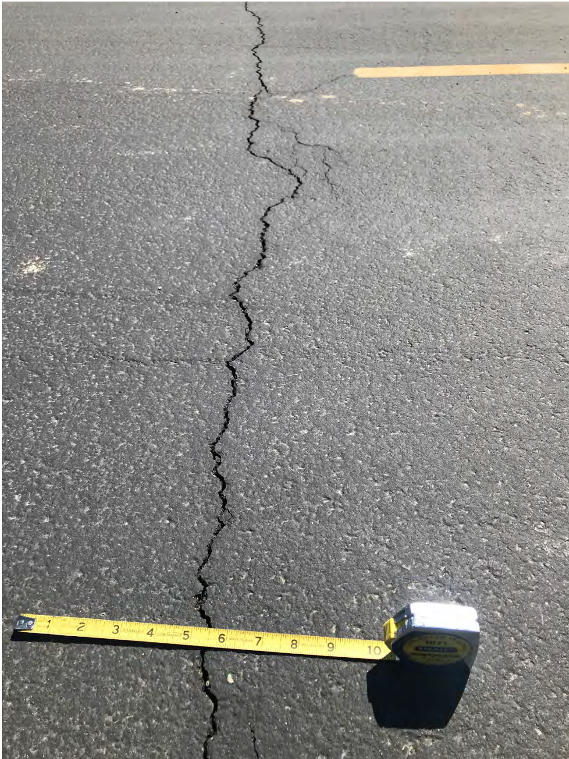
Loop Path System past half way toward La Cholla Blvd, typ smaller unpatched crack with displacement of ~1/4"
