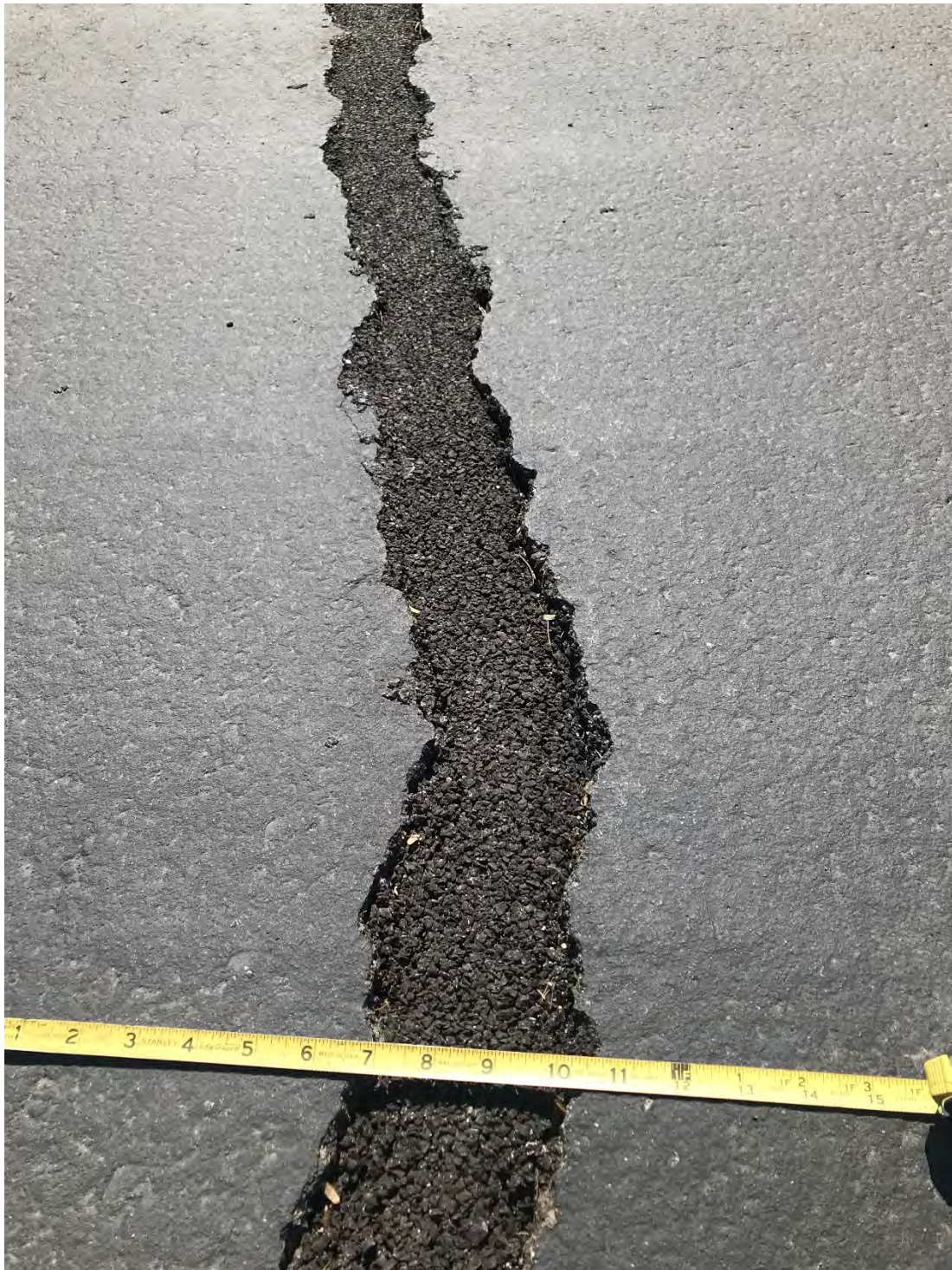
Loop Path System about half way between La Canada Dr and La Cholla Blvd, recently patched
