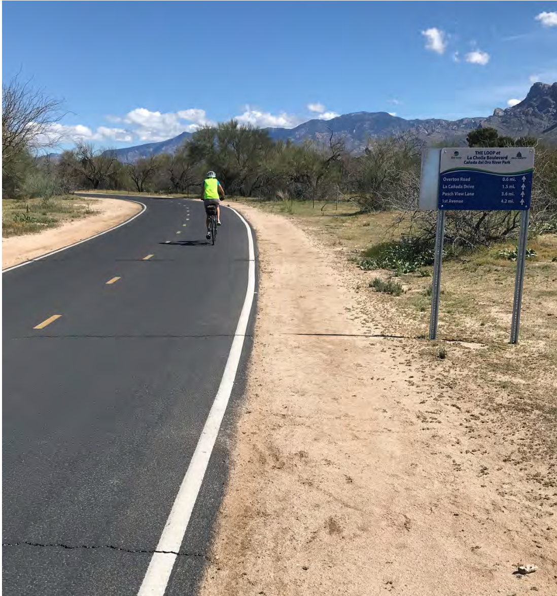
Loop Path System at La Cholla Blvd, looking back toward La Canada Dr, note typ crack frequency
