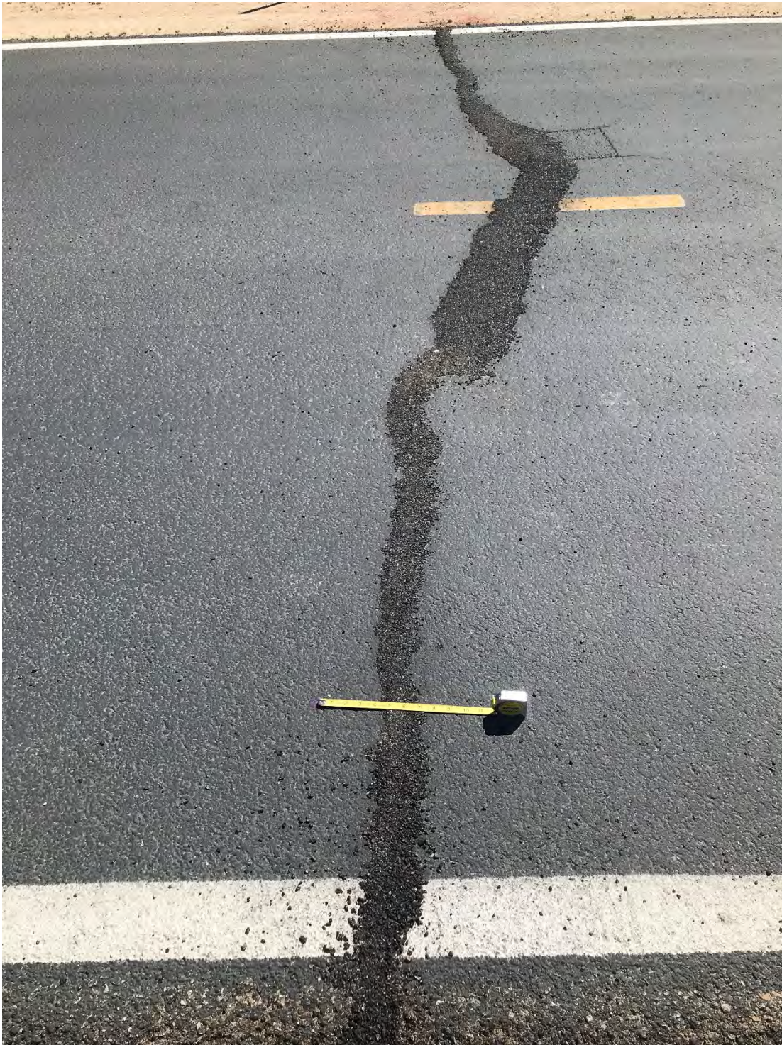
Loop Path System approaching La Cholla Blvd, typ crack recently patched
