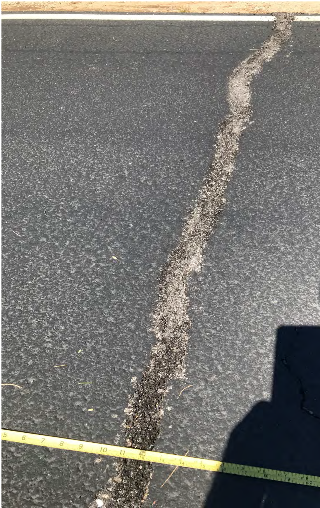
Loop Path System near La Canada Dr – typical crack, recently patched, note typ displacement
