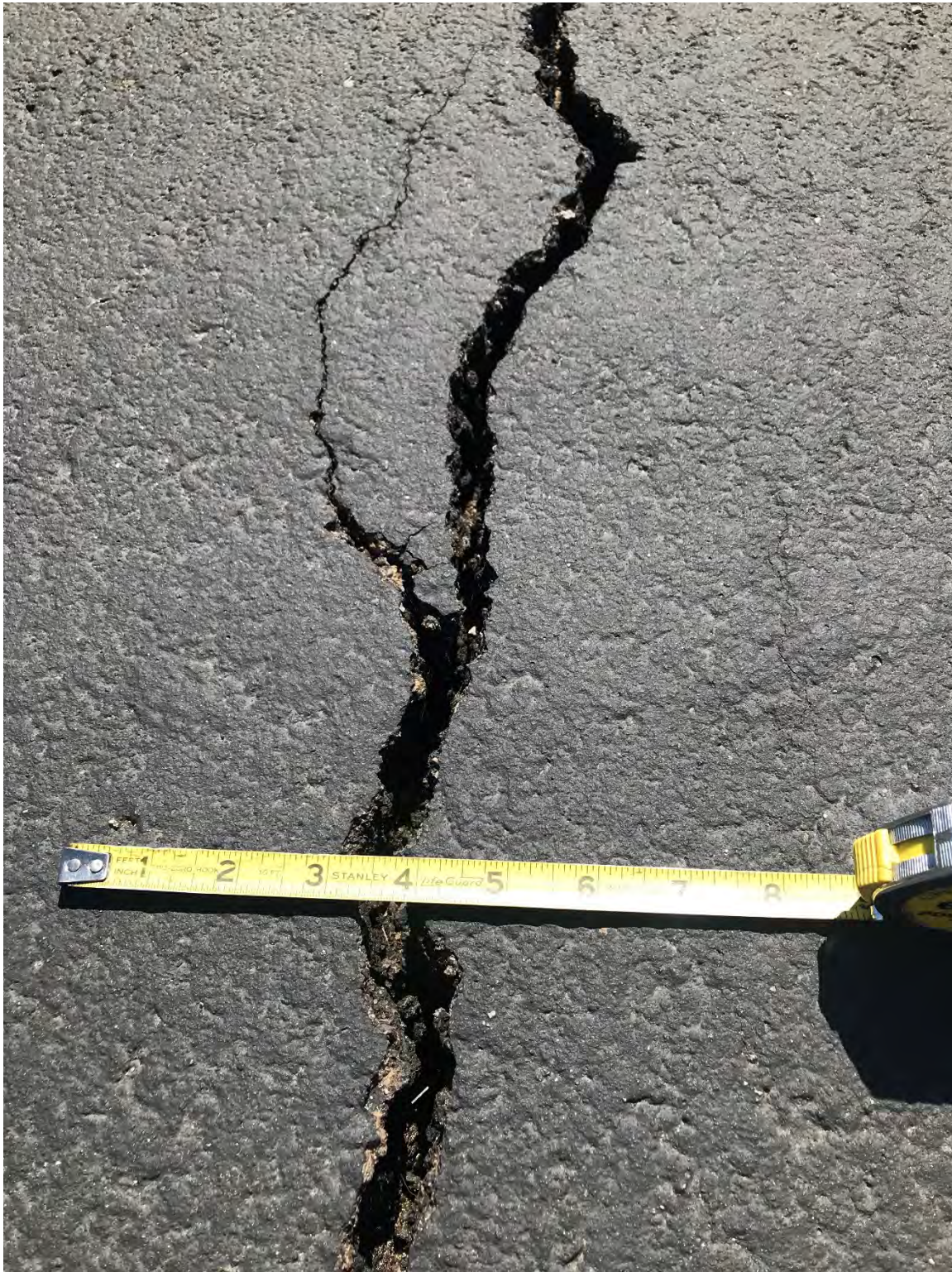
Loop Path System near La Canada Dr – typical crack, unpatched as smaller, note displacement
