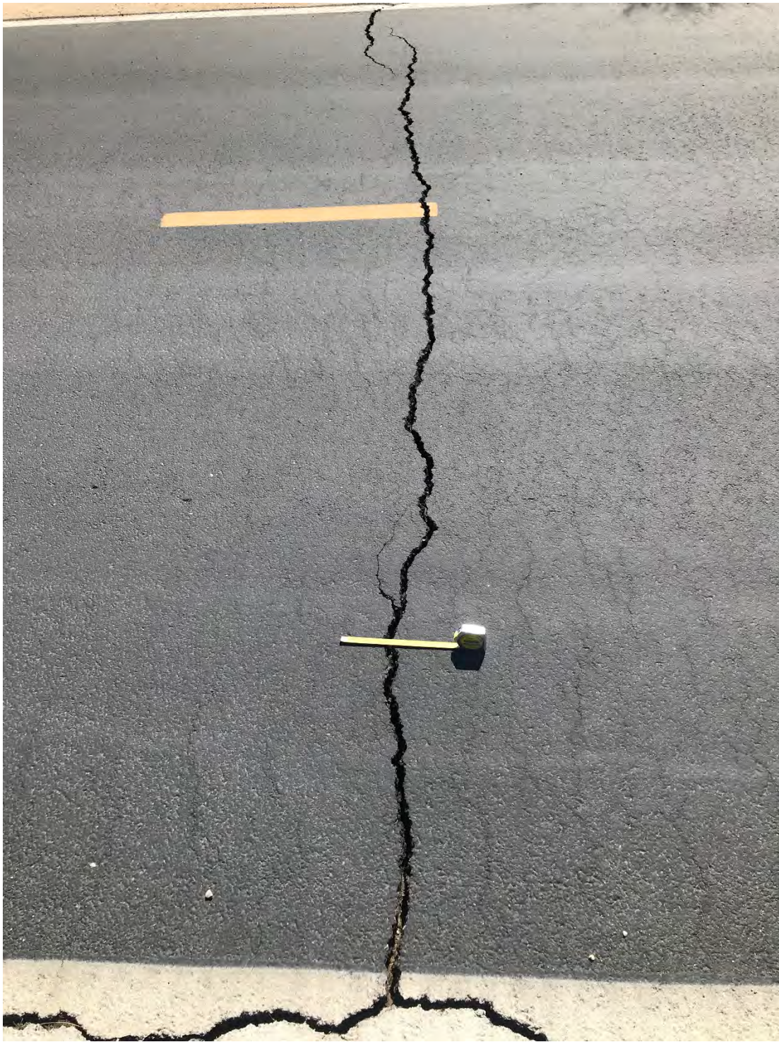
Loop Path System near La Canada Dr – typical crack, unpatched as smaller, note typ displacement
