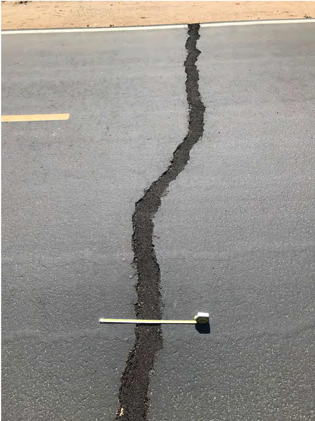
Loop Path System near La Canada Dr – travelling back toward La Cholla, typ crack recently patched
