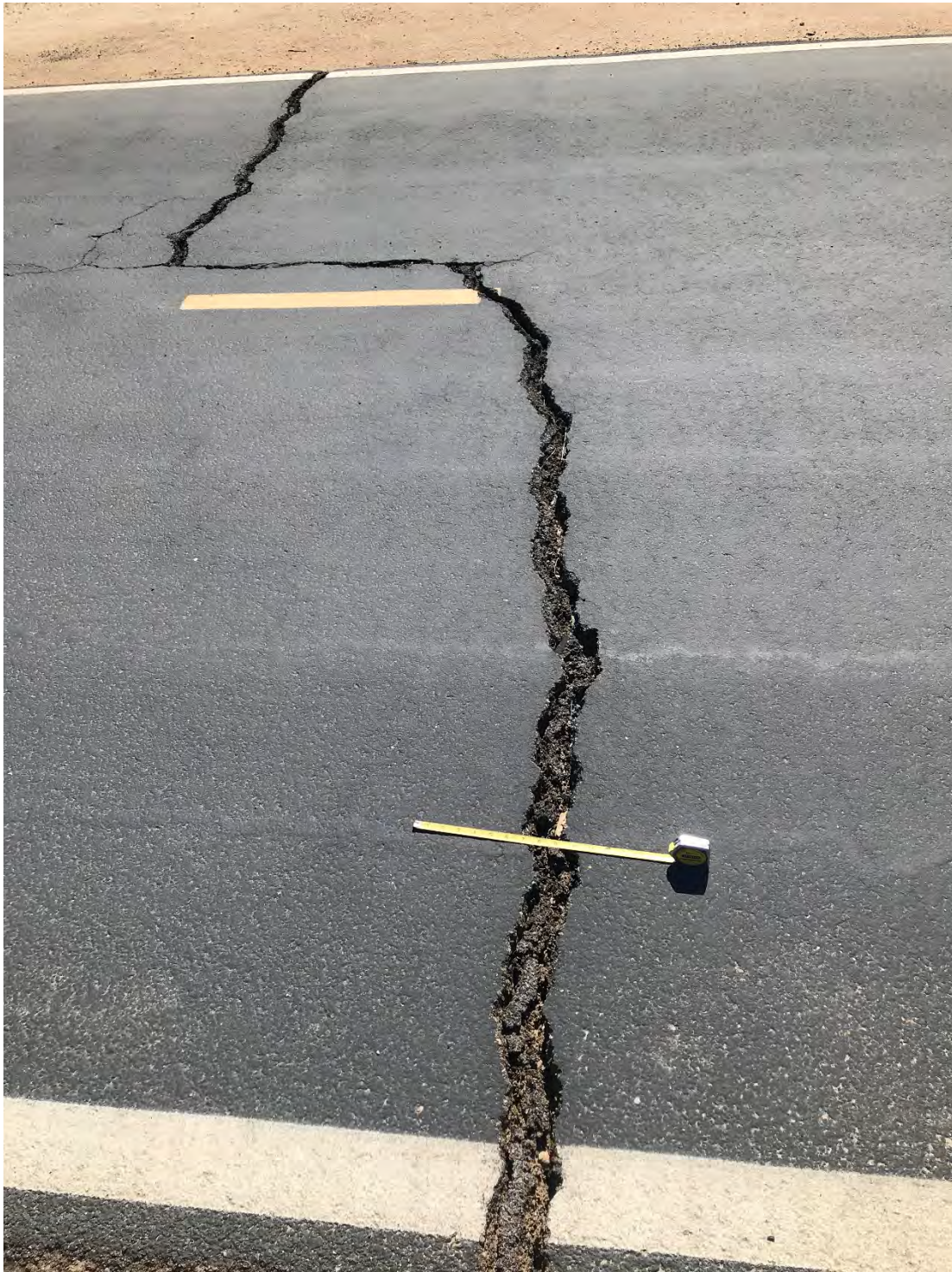
Loop Path System near La Canada Dr – travelling back toward La Cholla, typ crack, previously patched
