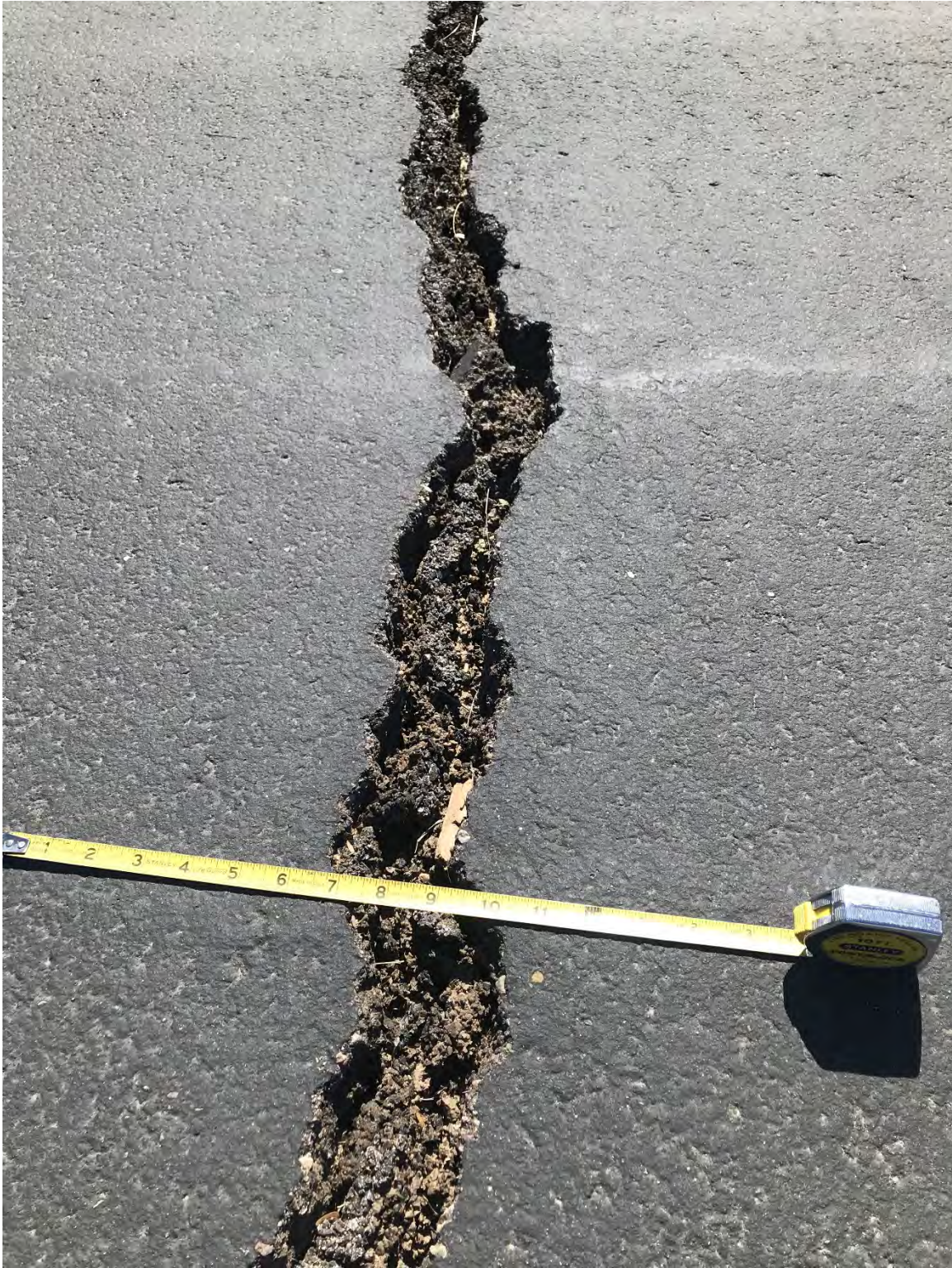
Loop Path System near La Canada Dr – travelling back toward La Cholla, typ displacement, previously patched
