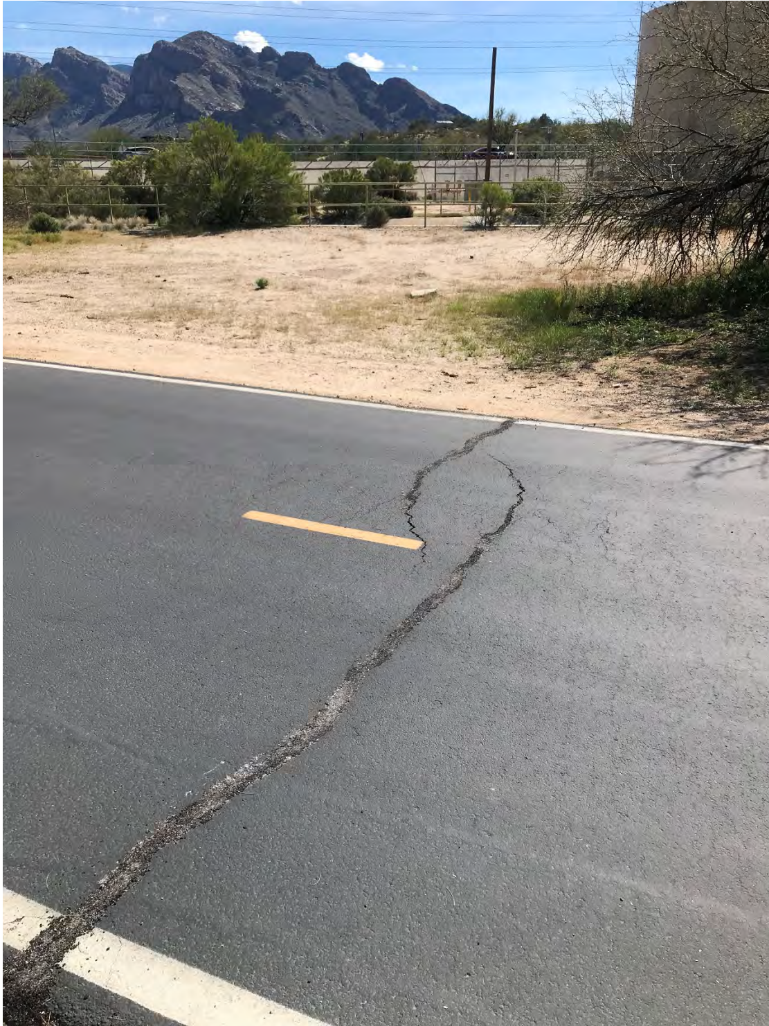
Loop Path System near La Canada Dr – typical crack, recently patched
