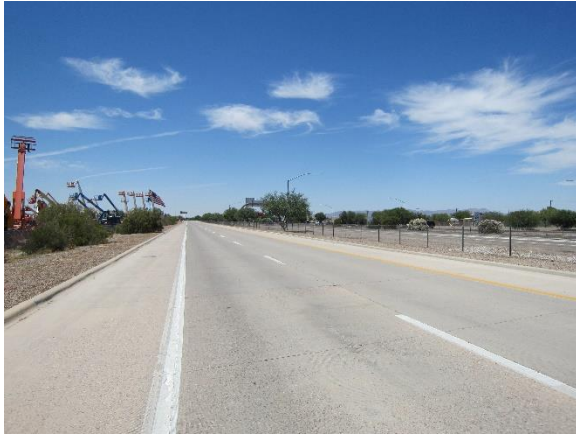
Street scene looking north along the I-10 Frontage Road
