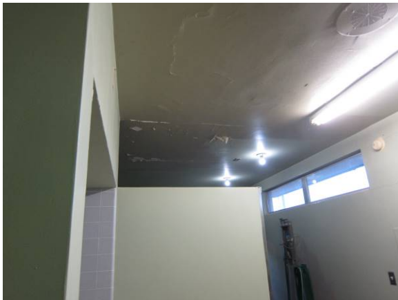
Ceiling damage in wash and grooming area
