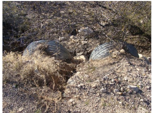
Dual Pipe Culverts West of Enclave Place
