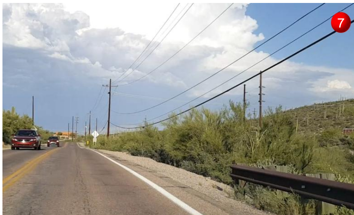
Fill slope concern beyond existing barrier limit.
