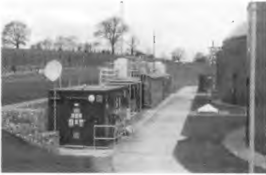
DMT Carborex® MS in the UK, 1500 SCFM raw biogas upgrading for gas grid injection
