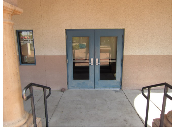
Faded exterior door paint
