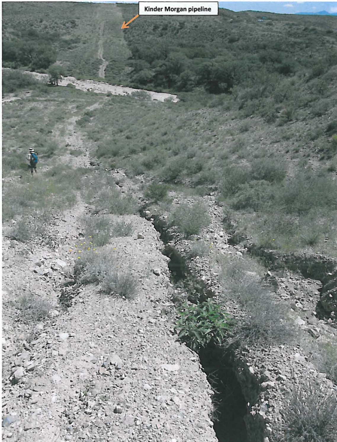
(Photo 3) Summer 2013. Cienega Creek/ Davidson Canyon. Pipeline built in 2007. Note deep erosion and evidence of off-road vehicle use that precludes any effective re-vegetation and habitat restoration.
