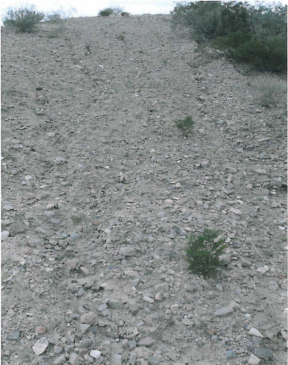
(Photo 8) Winter 2014. Cienega Creek/ Davidson Canyon. Pipeline constructed 2007. Note lack of top soil and erosion channels near crest of hill.
