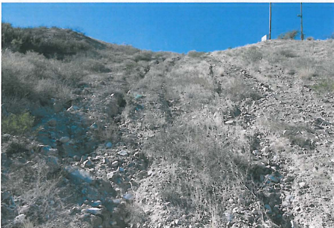
(Photo 7) Winter 2014 Cienega Creek. Pipeline constructed 2007. Close-up of erosion channels.
