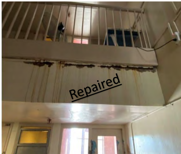
Upper tier steel railing rusted
