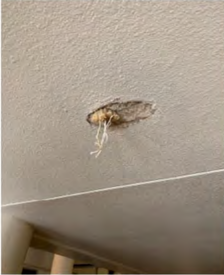
Water Damage - Ongoing Leak
