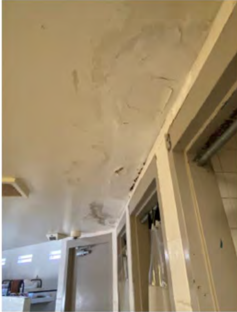
Damage from 2nd Tier Shower Leaks
