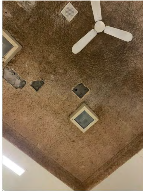
Falling Acoustic Tiles
