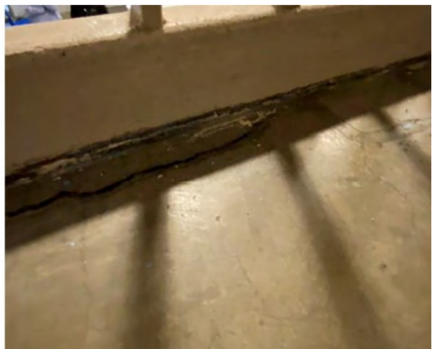
Broken concrete
