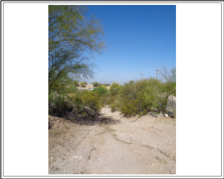
EXAMPLE OF THE EASEMENT ALONG THE NORTHWEST PORTION OF THE SUBJECT PARCEL
