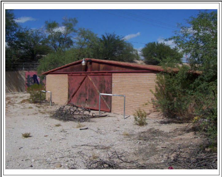
VIEW OF ACCESSORY BUILDING. PHOTO OBTAINED THROUGH COUNTY. 40' X 50' PRIOR STABLE
