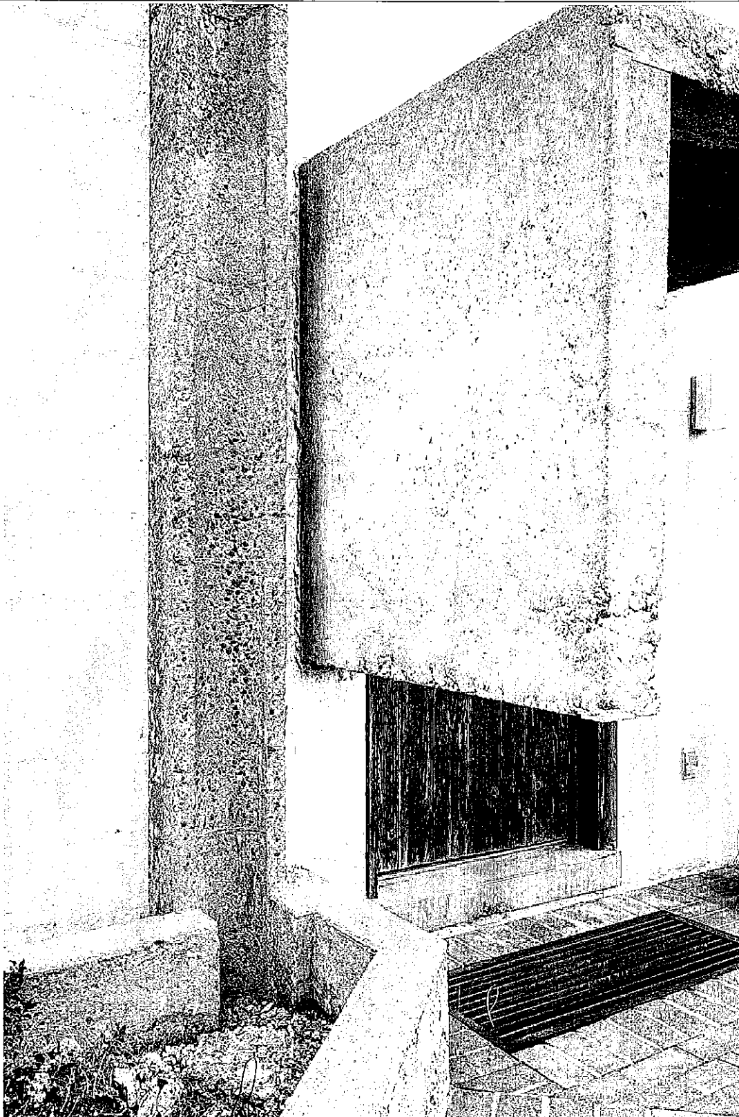
Photograph 14. Looking northwest, concrete shade system and concrete downspout.
