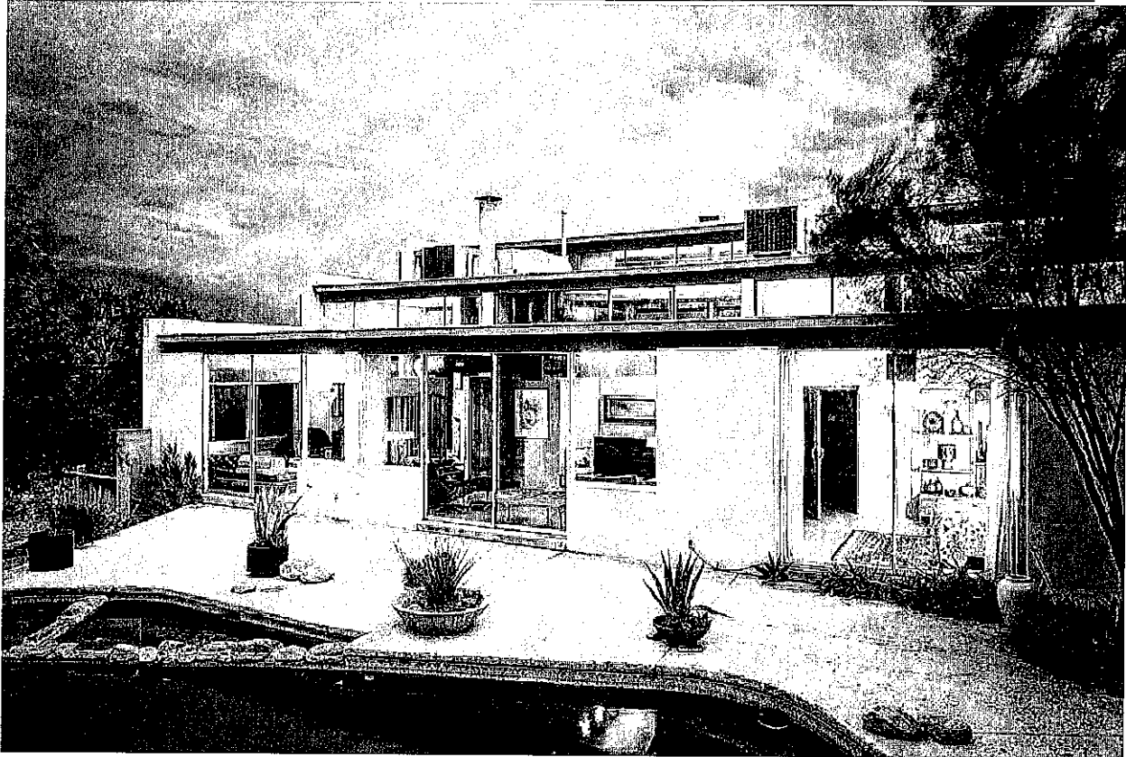
Photograph 3. Looking southeast, north facade.
