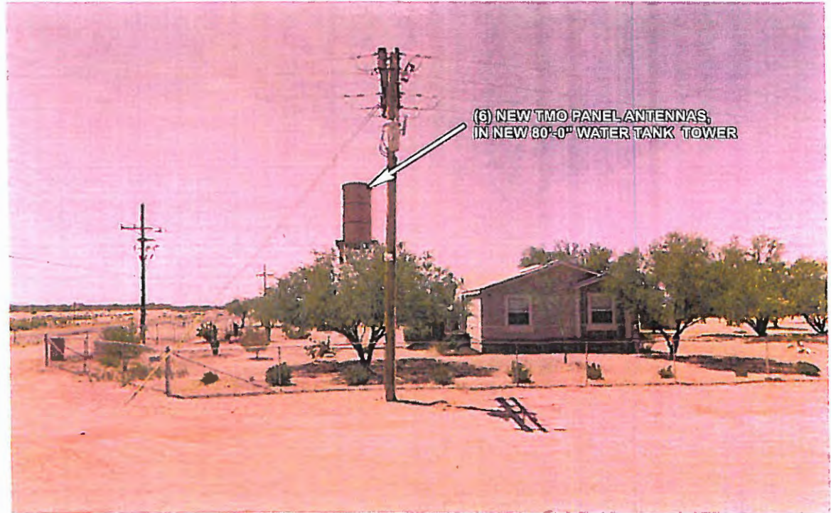
NORTH ELEVATION (LOOKING SOUTH)
