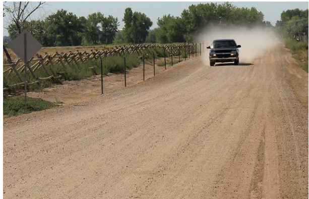
Figure 41. Photo. Dusty when dry.
