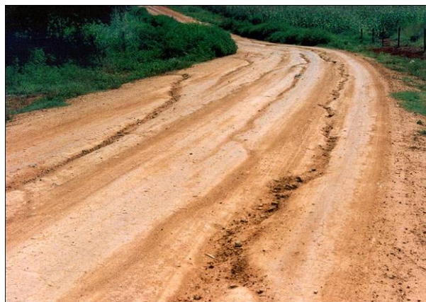
Figure 37. Photo. Longitudinal erosion.
