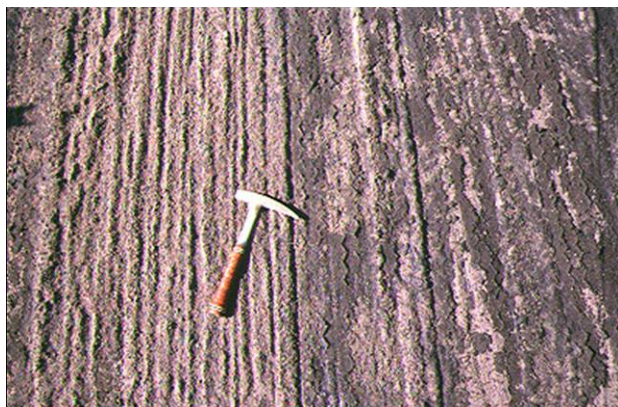
Figure 71. Photo. Poor penetration without pre-wetting.
