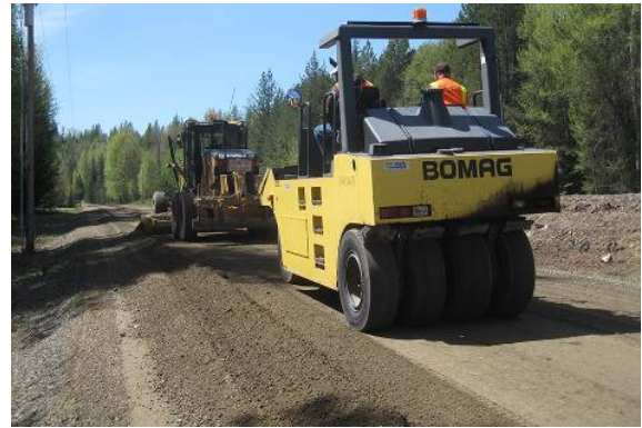
Figure 80. Photo. Compaction with rubber-tired roller.
