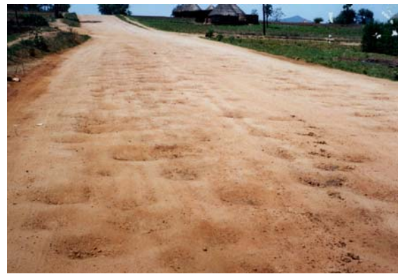
Figure 23. Photo. Potholes caused by poor drainage.
