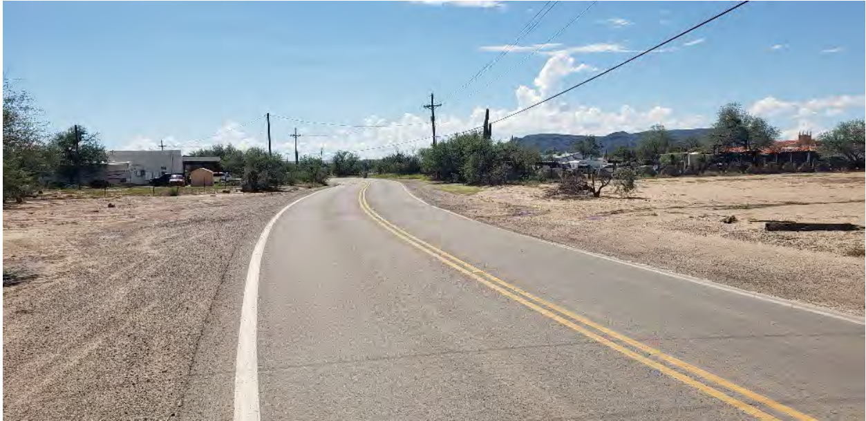
Looking North on Valley Indian Agency Connect Road. The project site is to the right.
