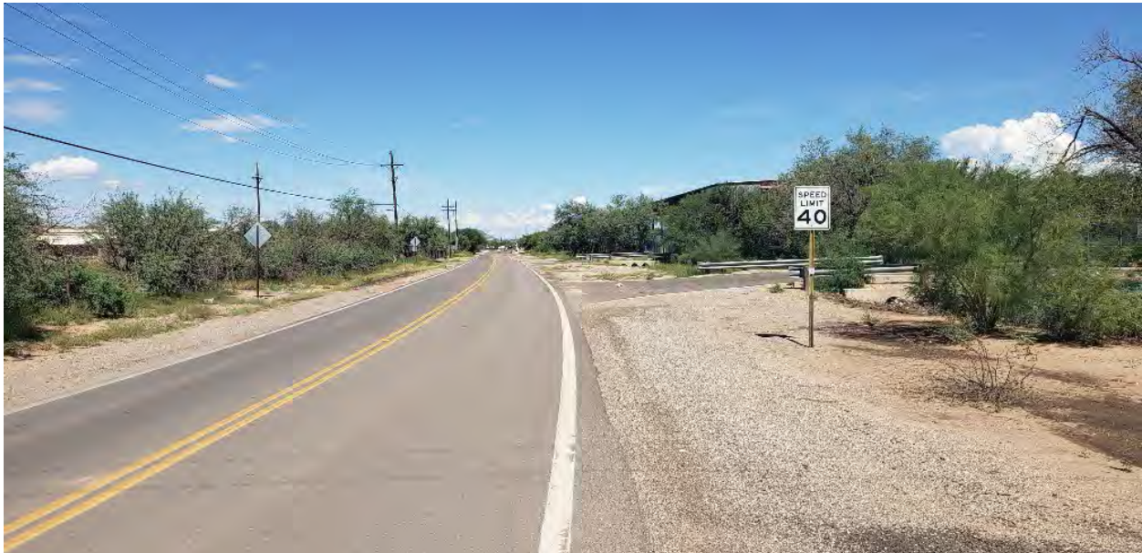
Looking North on Valley Indian Agency Connect Road. The project site is to the left.
