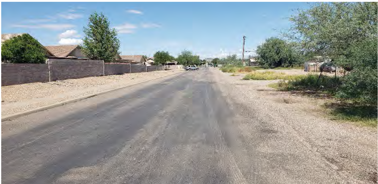
Looking North on Headley Road. The project site is to the right.
