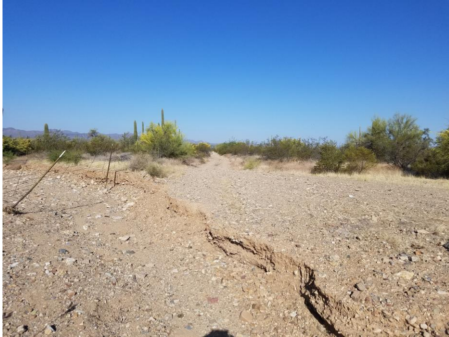
Sinagua Rd looking west (road partially washed out)
