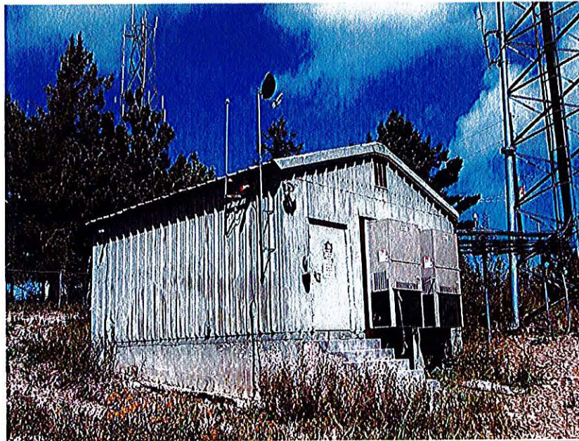
Facility #10 – Celco Partnership dba Verizon Wireless
