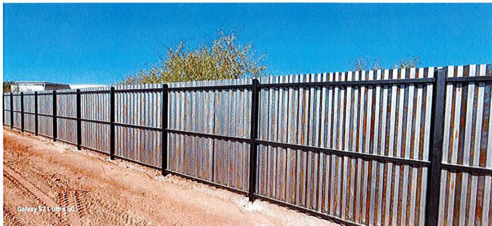
Example of the corrugated steel 6-foot wall/fence surrounding the property.
