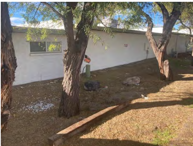
Units bedroom window look out on Dispensary.
