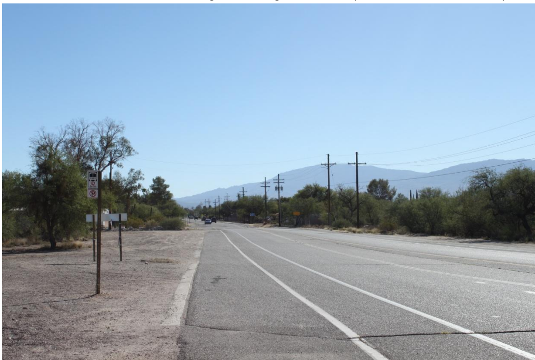
Near Southwest Corner of Site facing east along Cloud Road (uncurbed)
