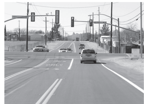
Drexel road to Country Club, under construction
