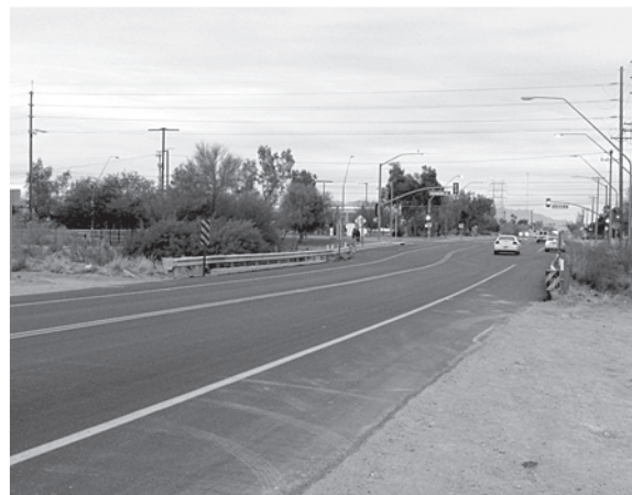
Country Club to Milber, under construction
