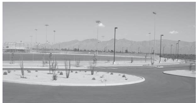
Lincoln Park Softball Field Improvements, completed
