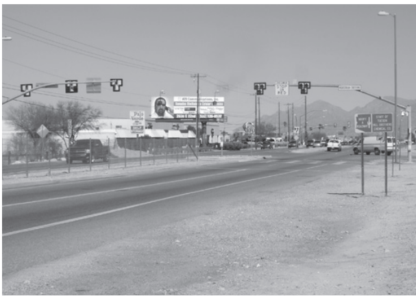
Palo Verde and Lincoln Hawk Signal and Crosswalk, under construction
