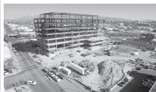
Downtown Court Complex, under construction
