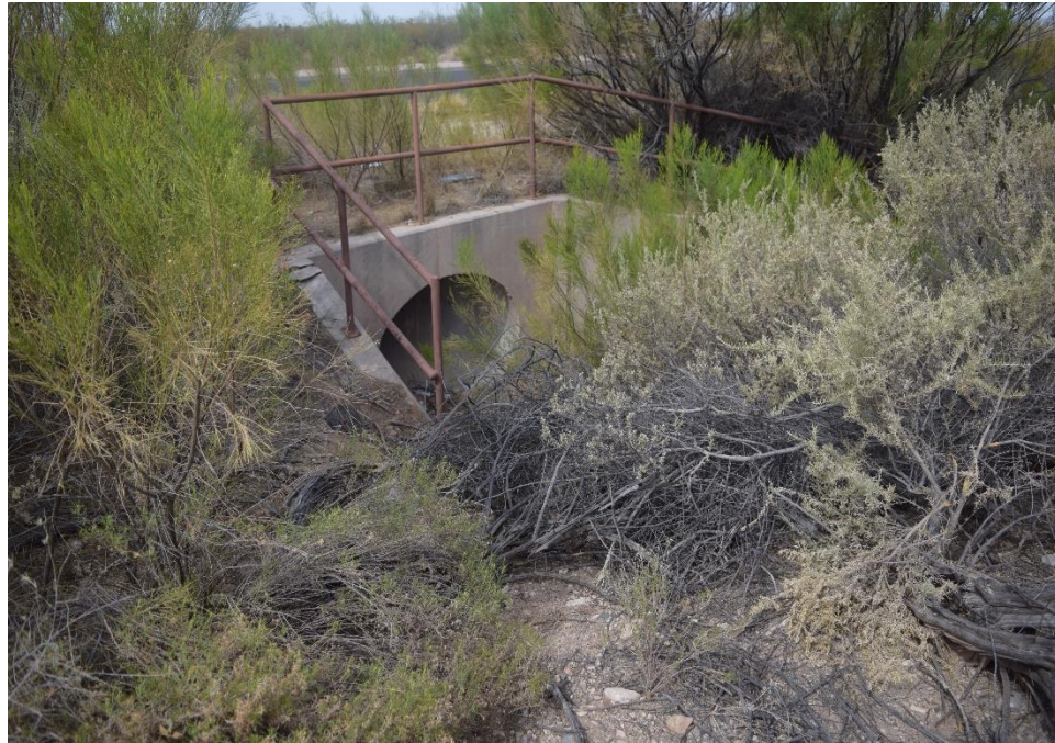
5) VIEW OF WASH/DRAINAGE COMING ONTO SOUTHWEST CORNER OF SITE
