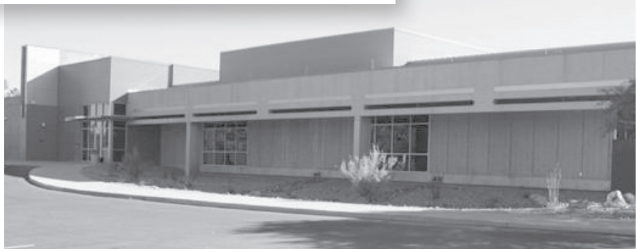
Pima Emergency Communications and Operations Center, completed
