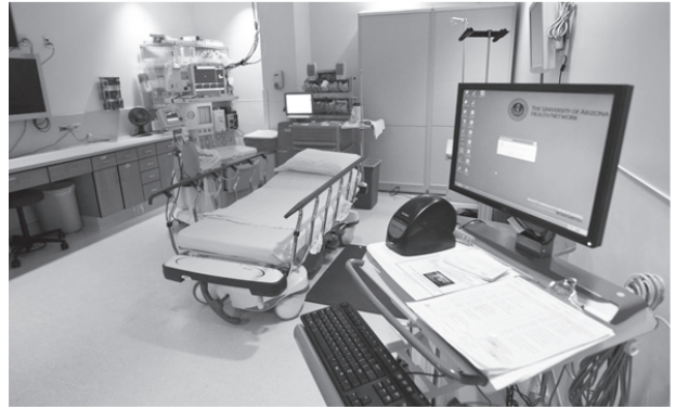
GI Lab at University of Arizona Medical Center South Campus, completed
