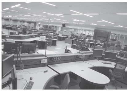
Pima Emergency Communications and Operations Center, dispatch area, completed
