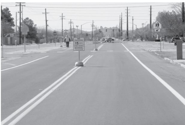
Drexel road to Country Club, under construction
