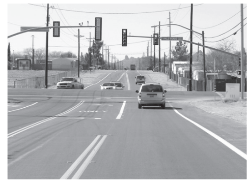
Drexel road to Country Club, under construction
