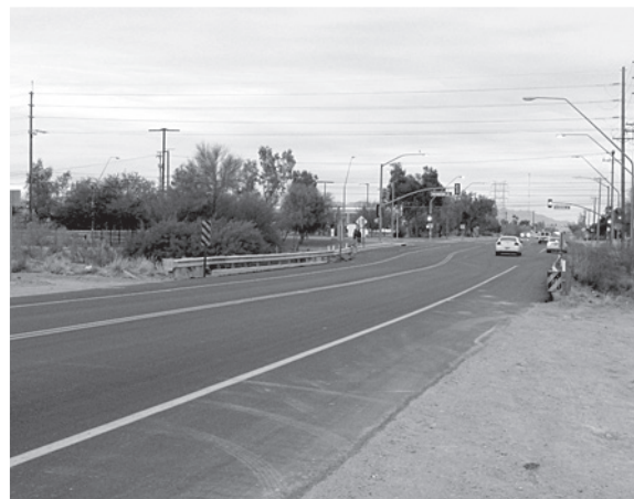
Country Club to Milber, under construction
