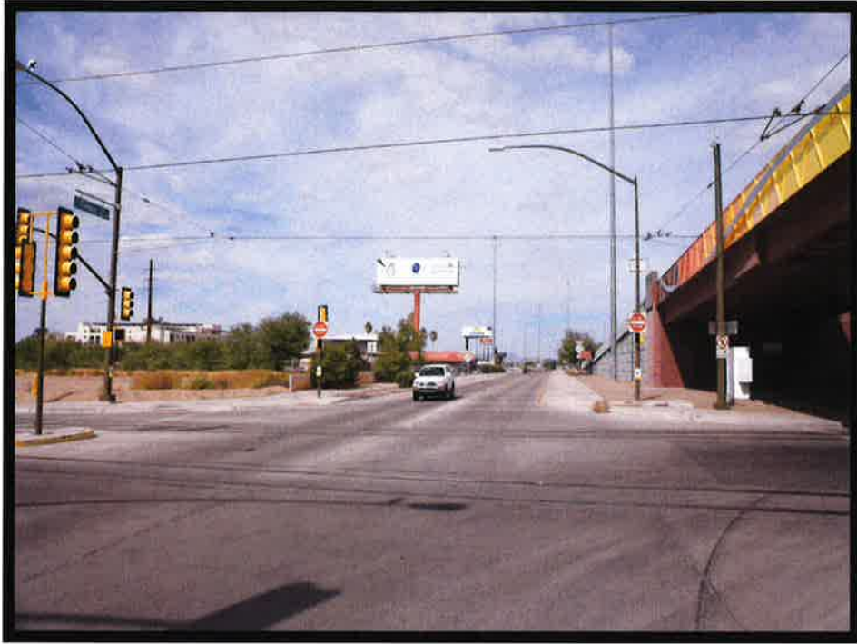
PHOTO 13 - VIEW NORTH ALONG FRONTAGE ROAD
