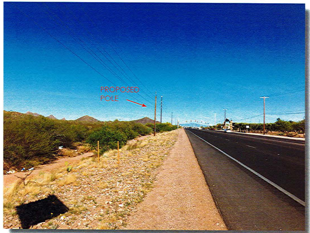
PROPOSED INSTALLATION OF NEW WOOD POLE, WITH ANTENNA AND ADDITIONAL EQUIPMENT ADDED TO POLE.
