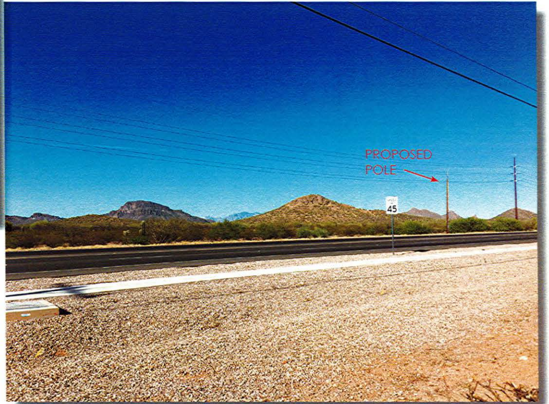
PROPOSED INSTALLATION OF NEW WOOD POLE, WITH ANTENNA AND ADDITIONAL EQUIPMENT ADDED TO POLE.
