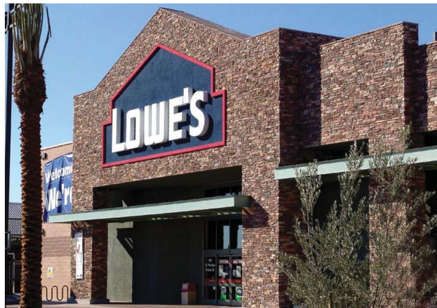
Old World Summerlin Blend Installed
