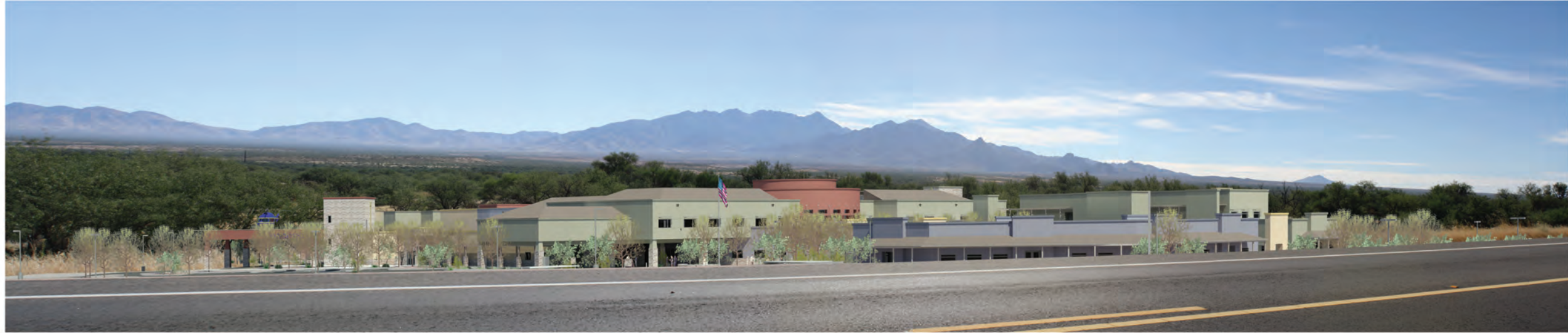
view from I-19 northbound
