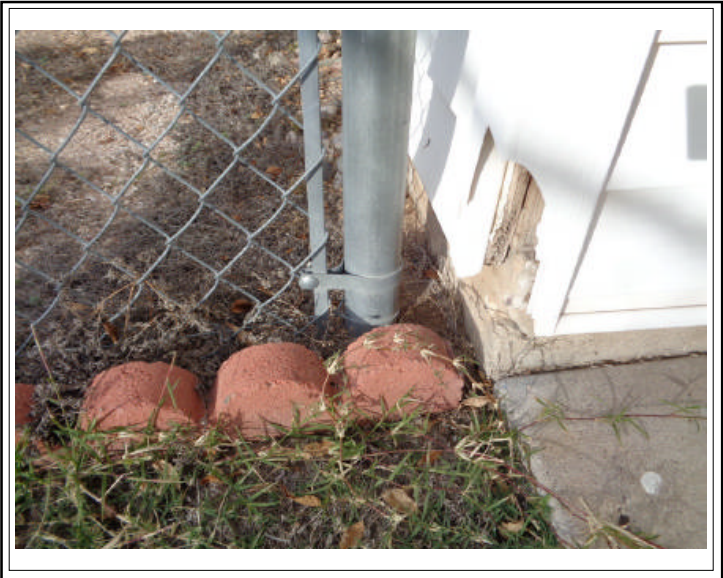
REFLECTS DAMAGED VINYL SIDING, AND EVIDENCE OF WOOD ROT
