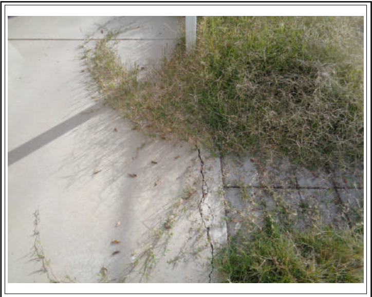
MINOR SLAB CRACK NOTED ON THE REAR PATIO
