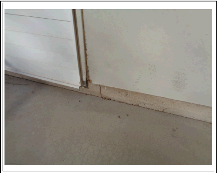
ADDITIONAL EVIDENCE OF TERMITE INFESTATION
