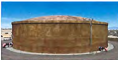
6.0 MG AWWA D110 Type III prestressed concrete tank recently completed for the City of Prescott by DN Tanks. We have built over 65 tanks in Arizona!
