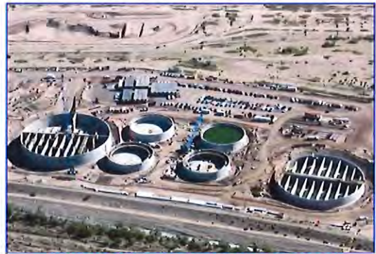
8.9 MG MBR and 5.1 MG chlorine contact chamber D110 prestressed concrete tanks constructed for Pima County
