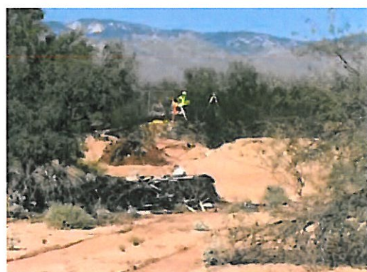
Photo 6, Worker surveying site for Meter Station.
