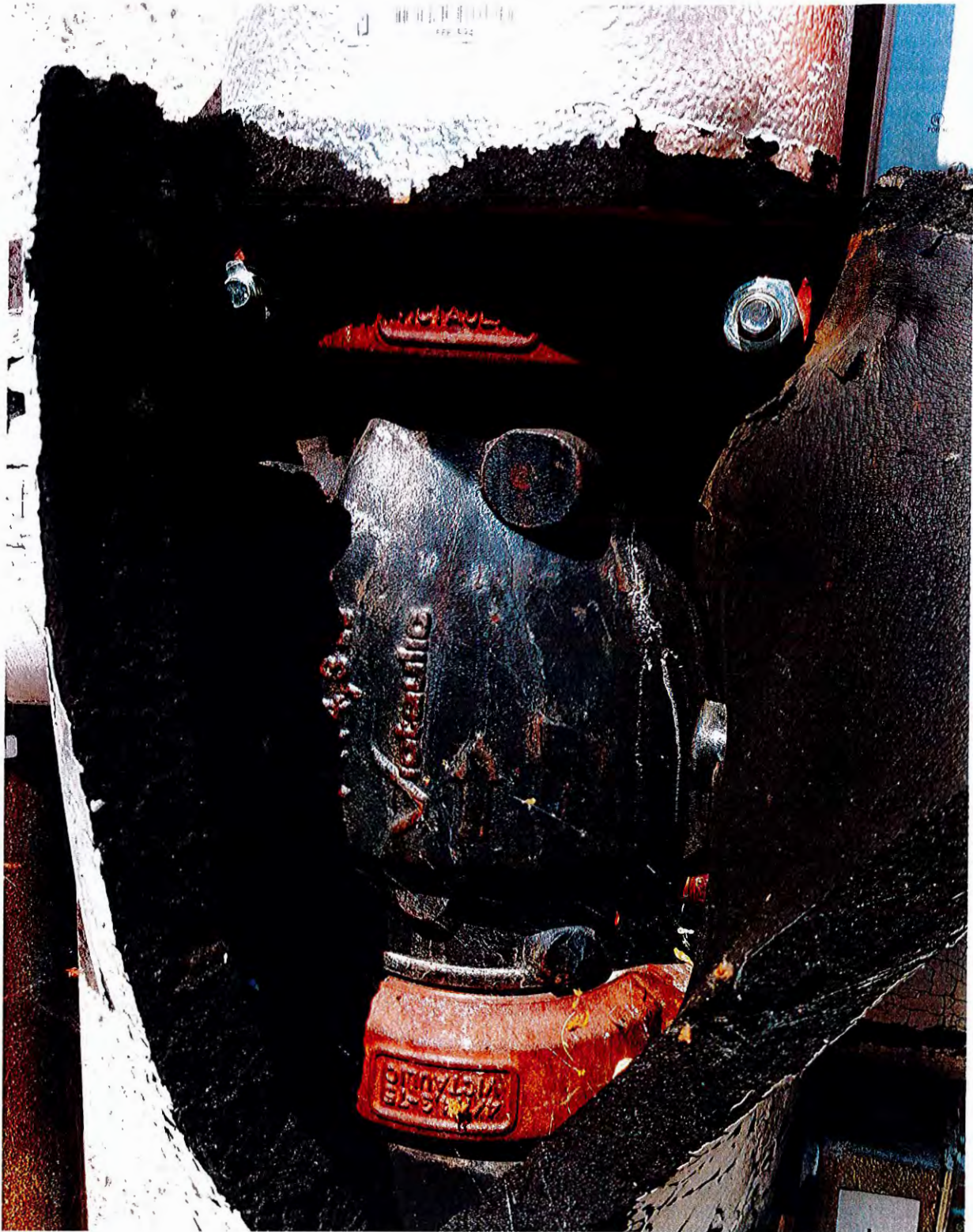
Photo of Item #12 Close Up of Fire Riser South End - Needs Attention
