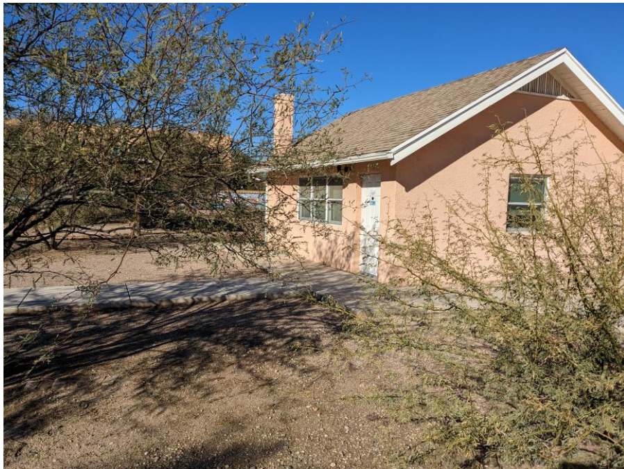
“Carriage House” Office (south and east elevations)
