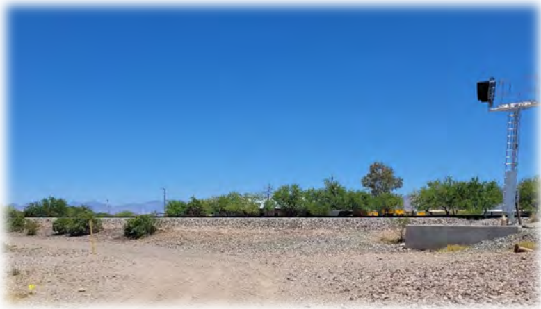
Raised UPRR tracks north of the property boundary.
