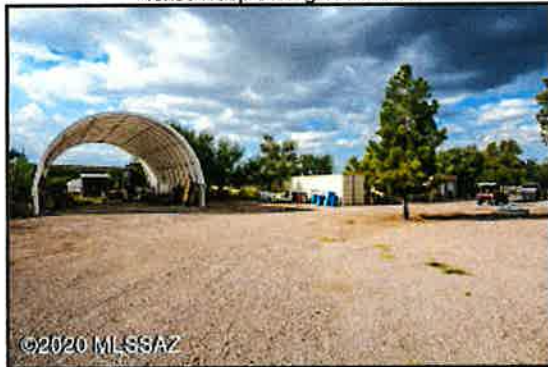
48x30 Hoop Storage Structure
