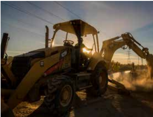
New Pima Animal Care Center under construction.
