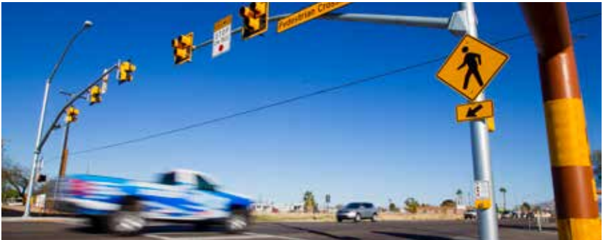
HAWK crossings on Palo Verde Road south of Drexel, completed in May 2016.
