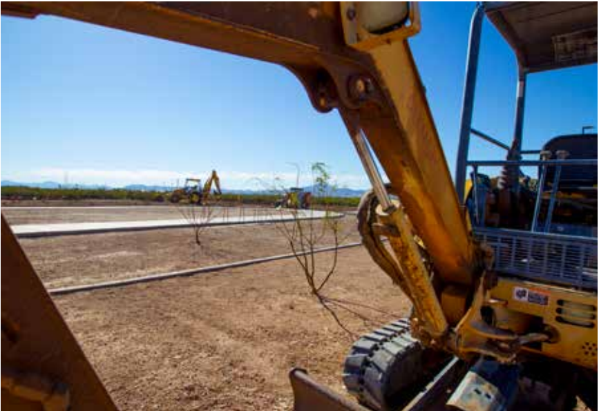
Southeast Community Park (Esmond Station) trail, under construction.
