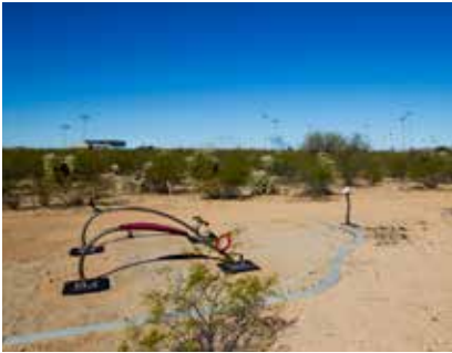
Southeast Community park, under construction.
