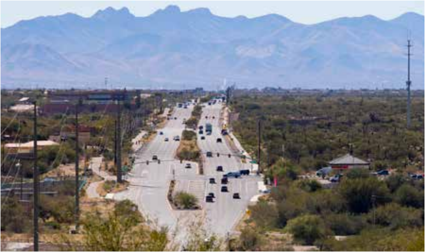
Houghton Road: Irvington to Valencia, completed June 2016.
