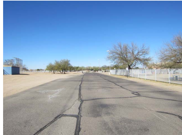
Photo 4: Street scene looking north
