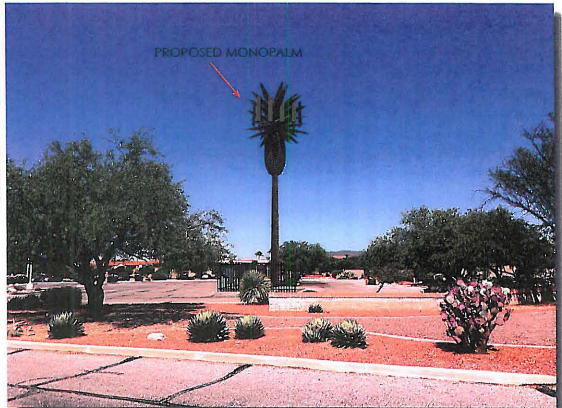
PROPOSED INSTALLATION OF A 58' MONOPALM WITH VERIZON ANTENNA ARRAY. ADDITION OF EQUIPMENT COMPOUND WITH CABINETS, UTILITY FRAME, AND GENERATOR, SURROUNDED BY AN 8' TUBE-STEEL FENCE. REMOVAL OF EXISTING CURB AND LANDSCAPING.
