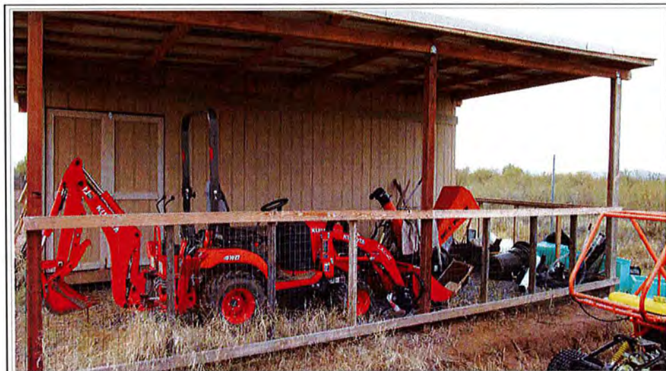
Workshop / Carport Building
