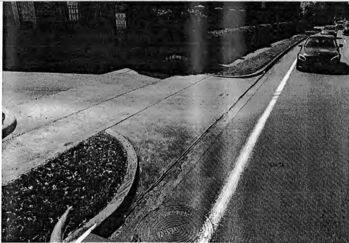
Drive Cut with Width Measurement
