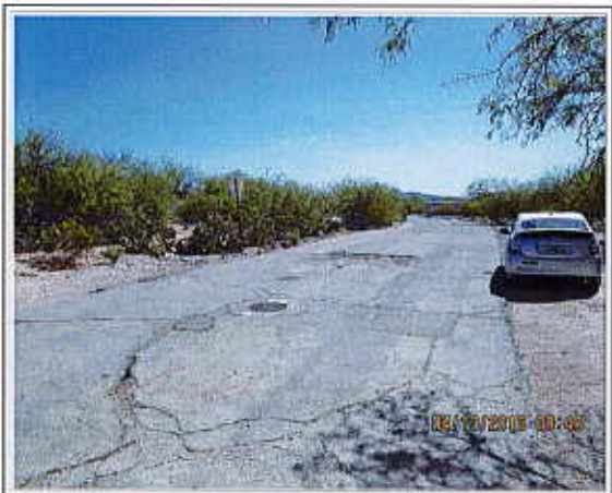
View East Along Indian Hills Road
