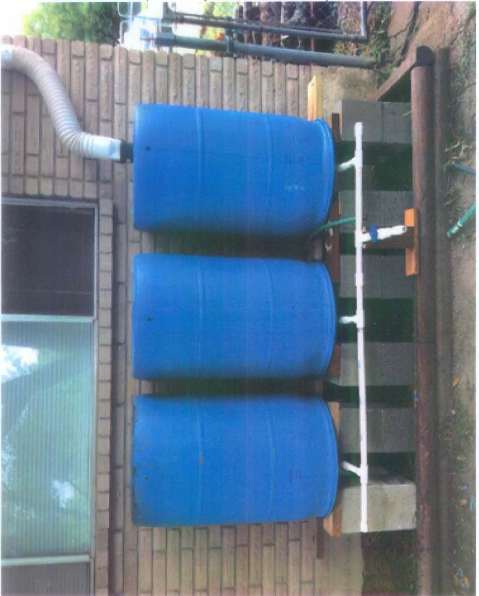
Three Cistern System (requires proposed screening if visible from street)
